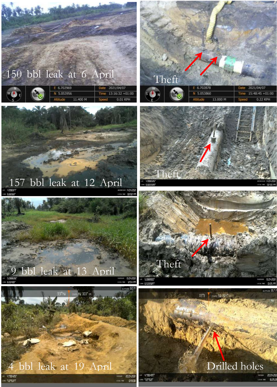
Figure 12: Oil spills caused by sabotage
