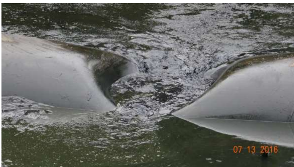
Figure 11: Close-up of spill point on 48” Forcados Export Pipeline at Ogulagha
