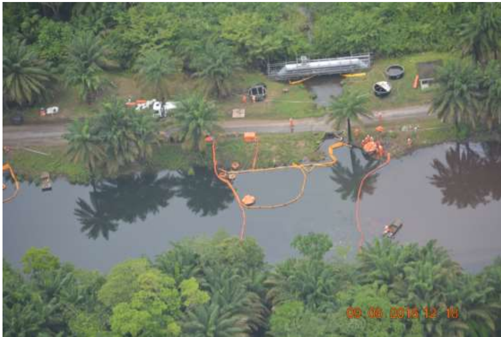
Figure 10: Part of spill impact on 48” Forcados Export Pipeline Right of Way at Ogulagha
